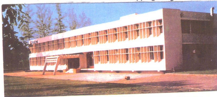
Manufacturing and Research & Development Centre, Navi Mumbai
