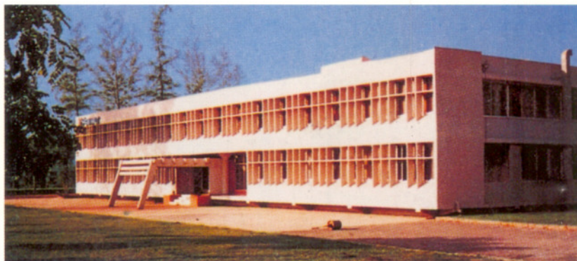
Manufacturing and Research & Development Centre, Navi Mumbai
