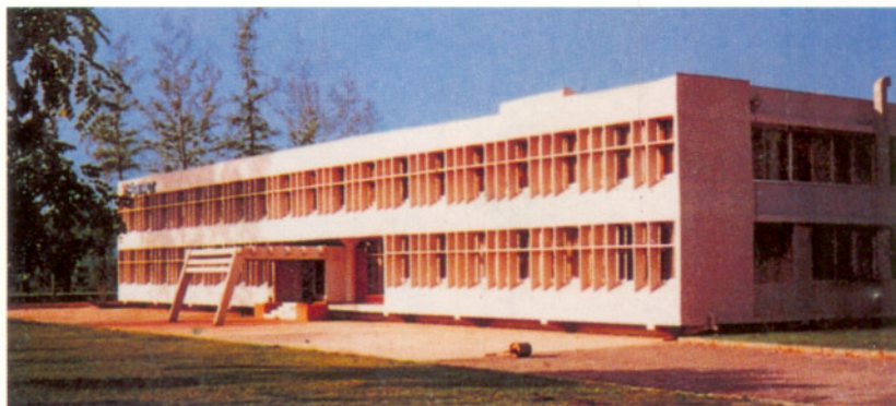
Manufacturing and Research & Development Centre, Navi Mumbai
